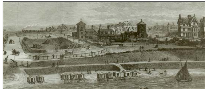
Westgate’s Tower Bungalows from the sea at St Mildred’s Bay - 1876 (Sea Tower is the Italianate-style detached villa to the left of the centre of the picture)
